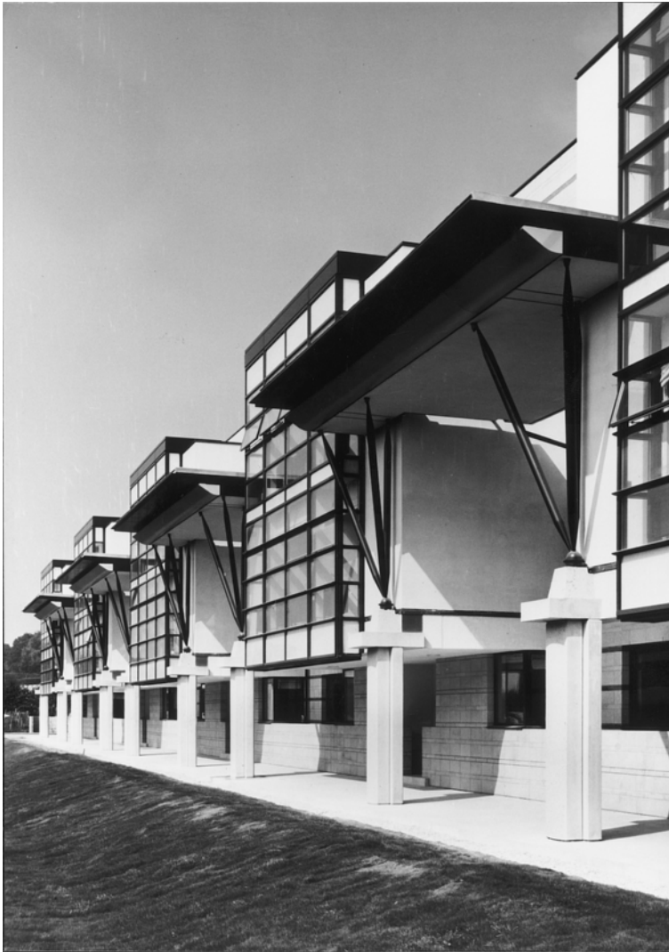
Figure 14.4 The 'great wall' of residential accommodation as actually built
